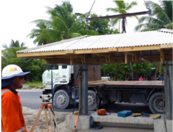
Bus shelter construction
