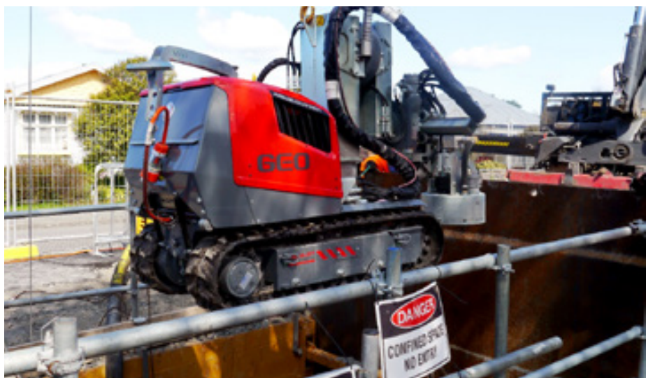
Geo the Robot lowered into the pipe for the first time
