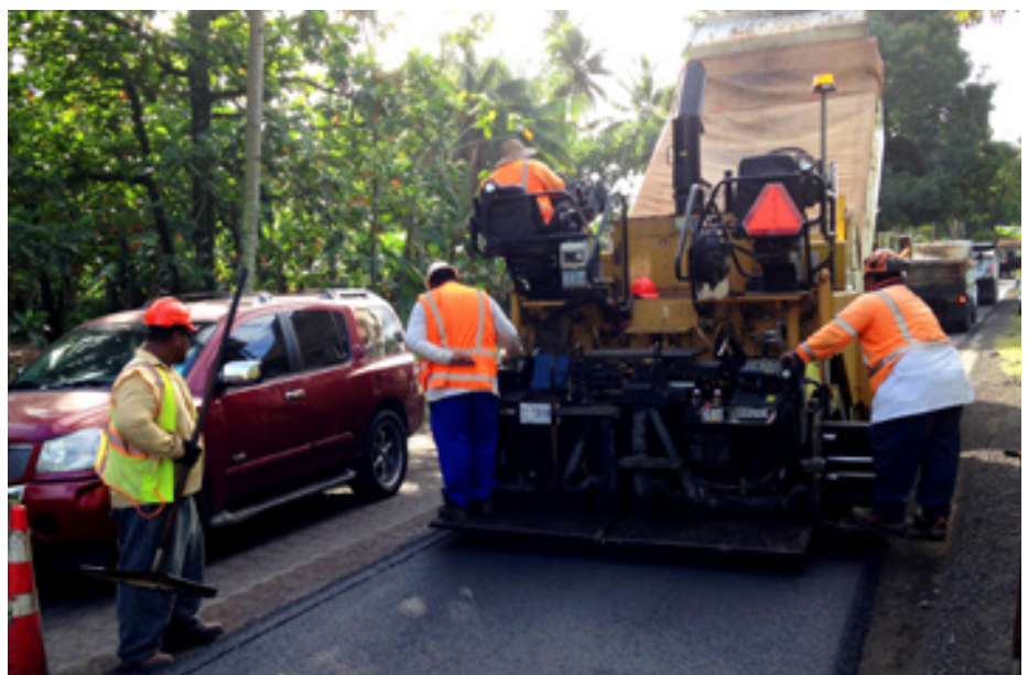
The asphalt surfacing was completed ahead of schedule and without incident
