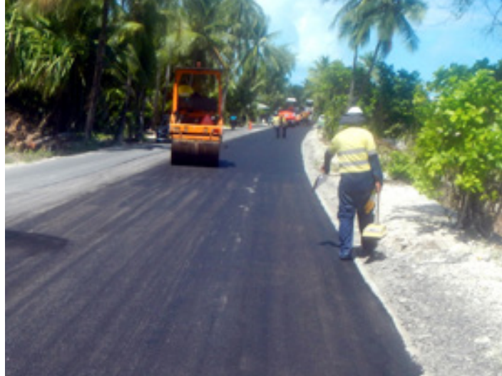
Asphalt to the main road
