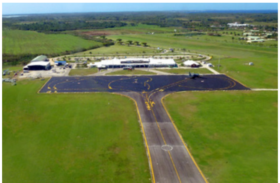
International Apron and Taxiway re-surfaced and re-lined
