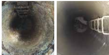
An asset before and after application of Milliken GeoSpray.
