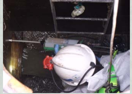
Technician fixing a leak by injecting through a manhole wall using a 'Quick Mix' cartridge system.
