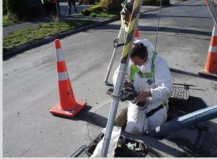
One of our technicians putting on their full face mask prior to repairing a leak in a manhole.
